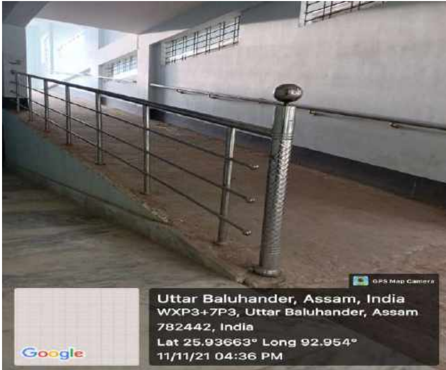
Ramp for Disable person for moving towards Class Rooms
